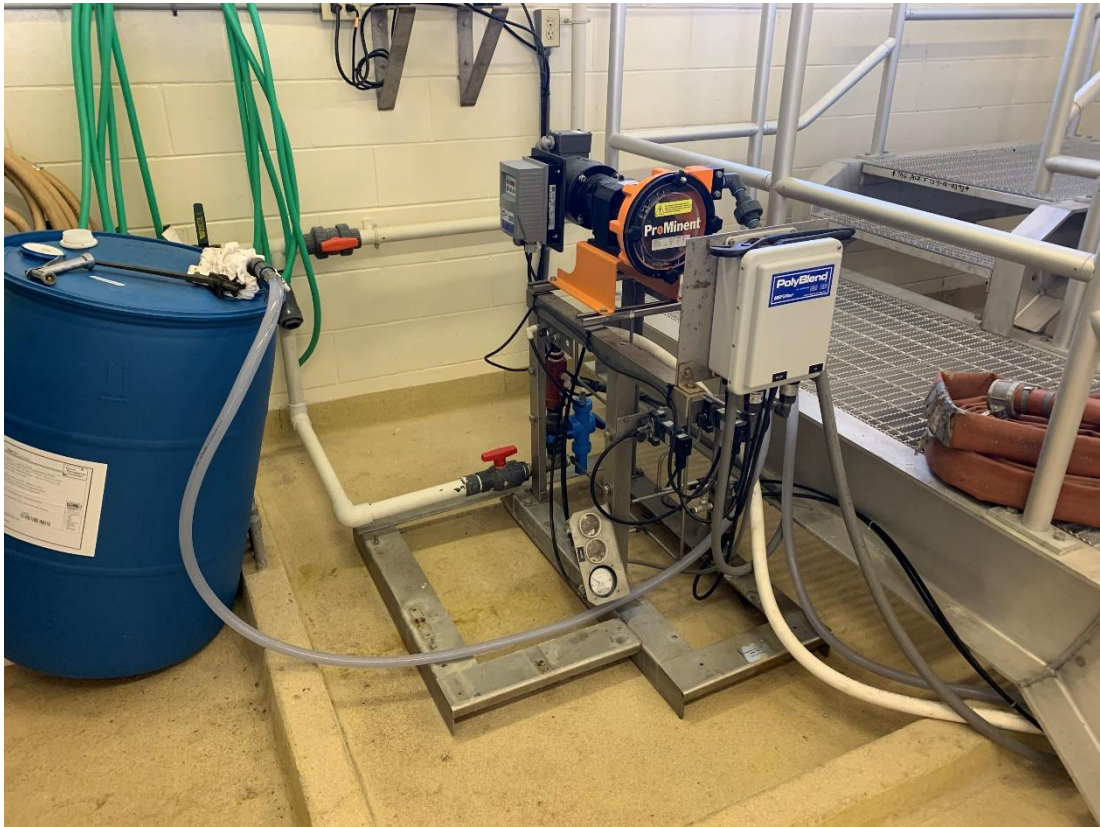
Photo 3 – Sludge Thickening System Polymer Feed System
