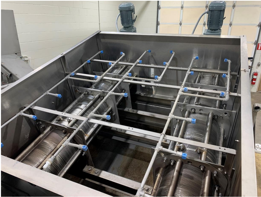
Photo 5 – PWTech Volute Press Dewatering Drums
