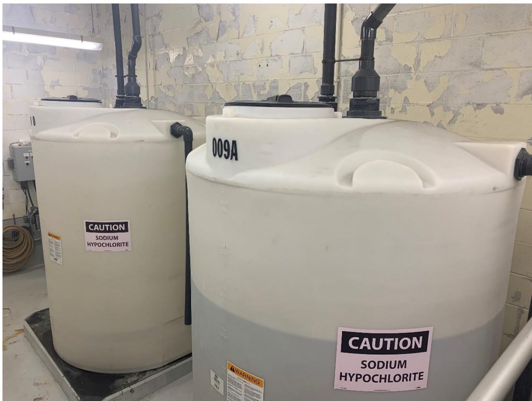
Photo 6 – Sodium Hypochlorite Storage Tanks
