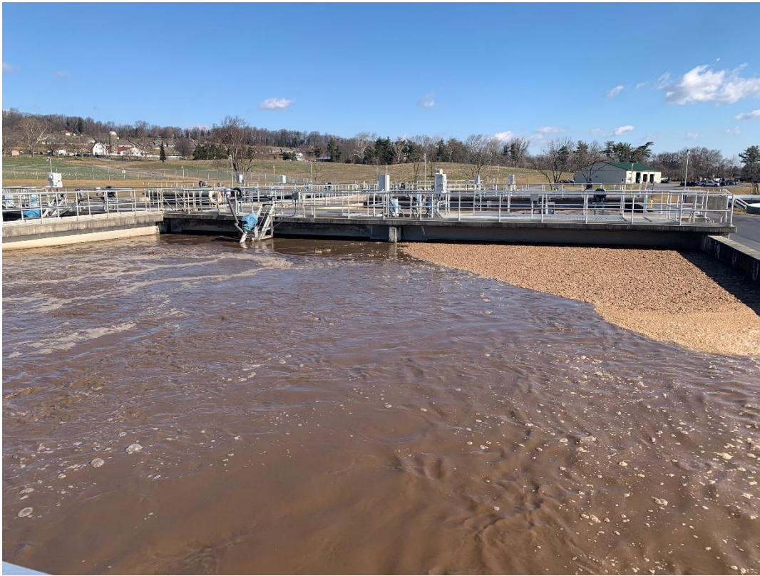
Photo 1 – Oxidation Ditch
