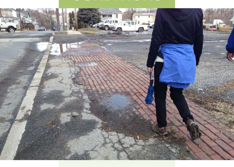
Broken asphalt and uneven bricks are present for a short section near the approach to the railroad tracks.
