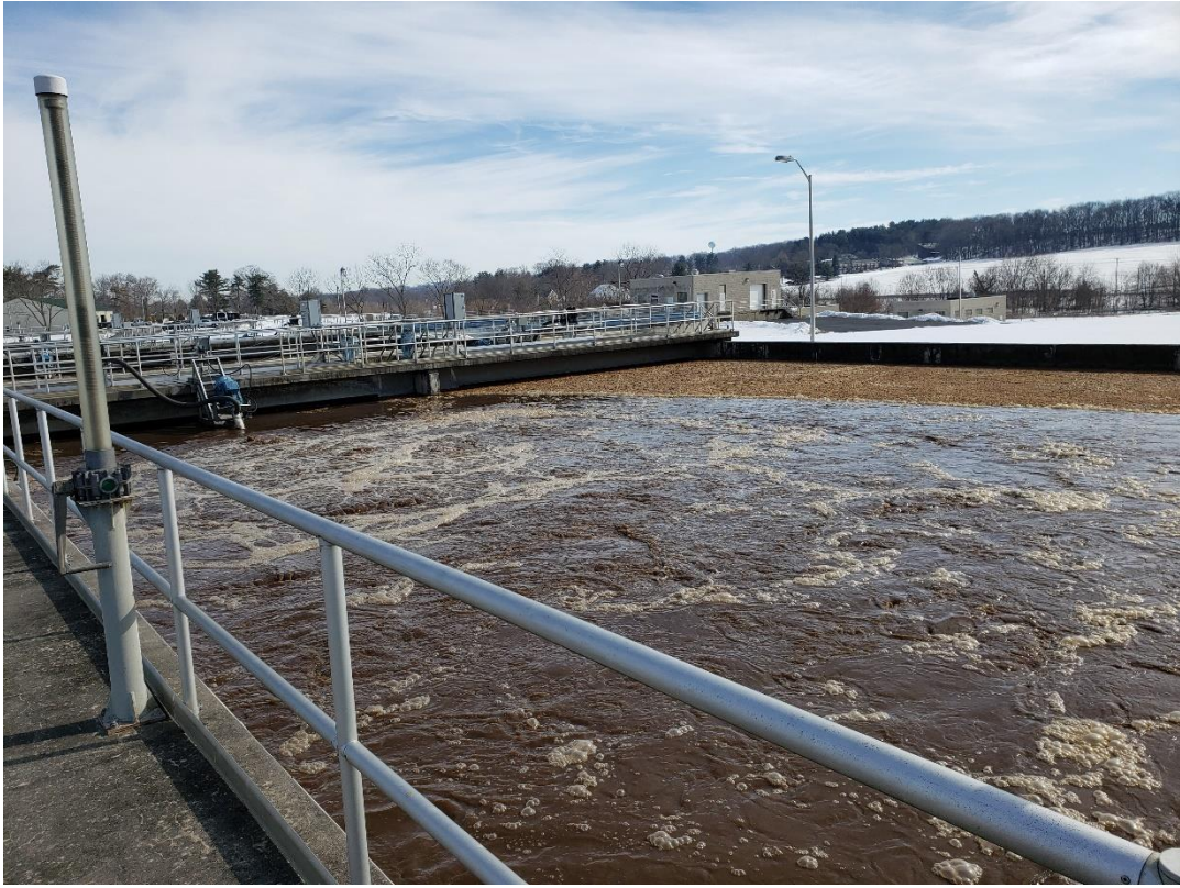
PHOTO 1 – Oxidation Ditch
