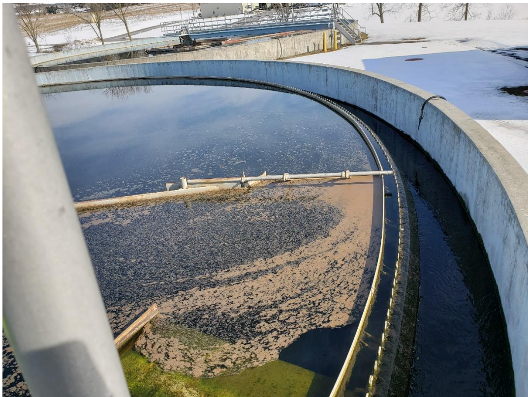
PHOTO 4 – Repaired Skimmer Blade on Clarifier No. 2
