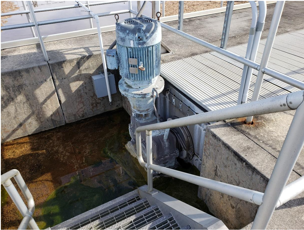
PHOTO 3 – Oxidation Ditch Rotor Drive and Assembly
