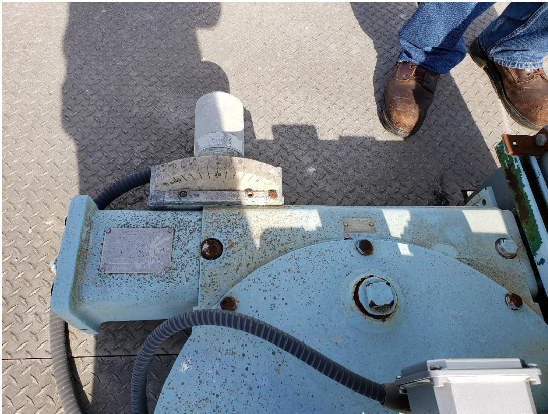
PHOTO 5 – Clarifier Drive Torque Overload Device
