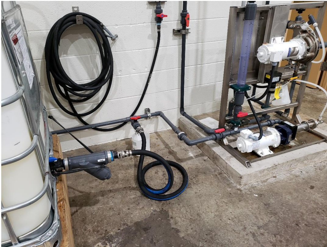
PHOTO 7 – Polymer Feed System in Dewatering Building
