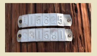
In order to provide PPL with the information they need to send out their service staff to the proper location, you should be prepared to provide the unique pole number from the street light pole. Each pole with a street light should have a small metal placard located at eye level on the pole containing a two-line PPL pole number. If you have any questions, please reach out to the Borough 717-367-1700.
